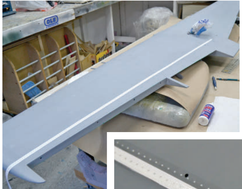
Above: Rivet tape is installed and ready for glue. A light bead of glue and a quick swipe to fill the holes, and you're ready to remove the tape to reveal an even line of rivets. Right: One set of rivets dries while the next is ready to have the tape removed.
