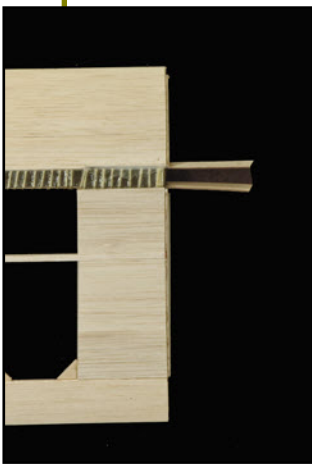
Double ribs "1" at dihedral break showing surface sheeting overlapping inner ribs only.
