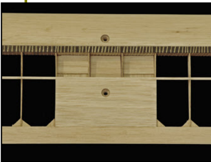
Finished mounting bolt holes showing relief for bolt heads in the upper surface sheeting.
